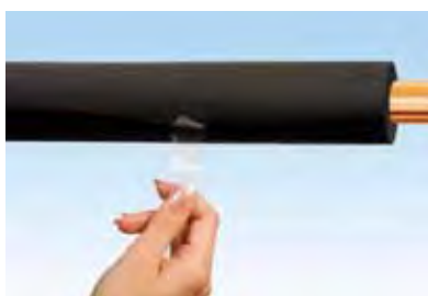
Peel release film from overlapping tape and bring over slit
