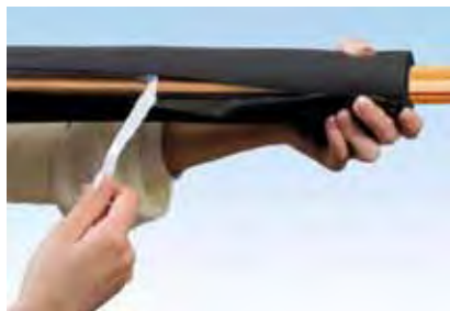
Peel inner release film
